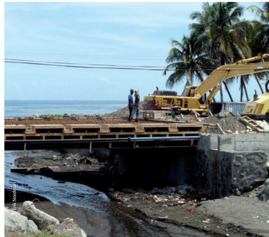
Workers rebuild a bridge that was destroyed in a storm.
